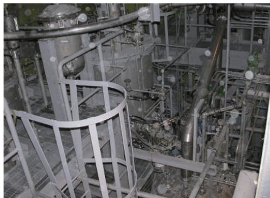
High Volume Reduction Solidification System for Wet Wastes in Kuosheng Nuclear Power Plant
